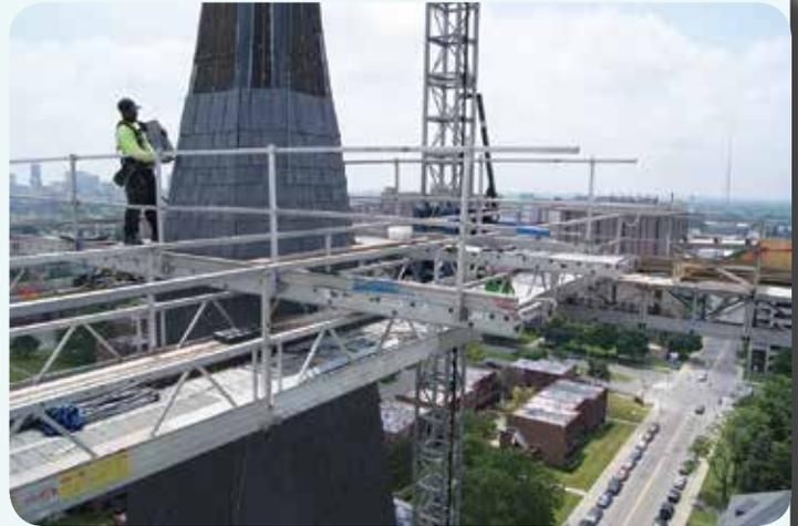
The Romanesque like 200' steeple at St. Josaphat's church was heavily damaged in a wind storm. As a result, the steeple was unstable and it became an urgent safety concern for the congregation, roads and for pedestrians below as the slate started to break off. For Detroit Cornice & Slate this was an opportunity to bring new life back to this much loved church.
