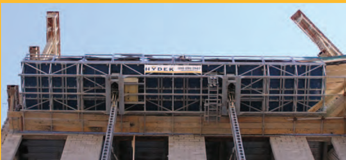
USE BRIDGES TO EXTEND THE WORK PLATFORM OUT TO 64 FT, IN 2.5, 4, OR 8 FT INCREMENTS
